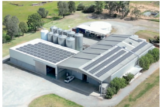
80kW nameplate capacity solar power system
