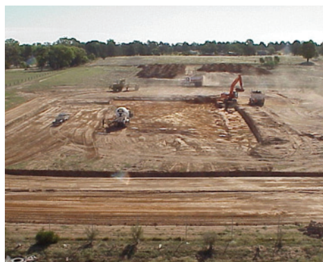
Earthworks in preparation for the BioAg Liquids Plant in Narrandera, March 2002.
